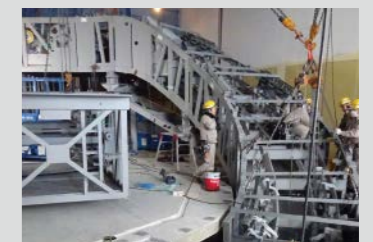
Truss installation work
