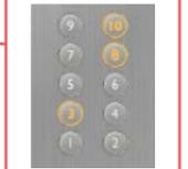
The destination floor has already been registered. The passenger does not need to press a floor button in the car.
